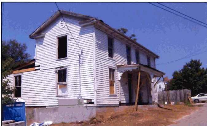
707-709 Fourteenth Street under renovation. Note the new foundation.
